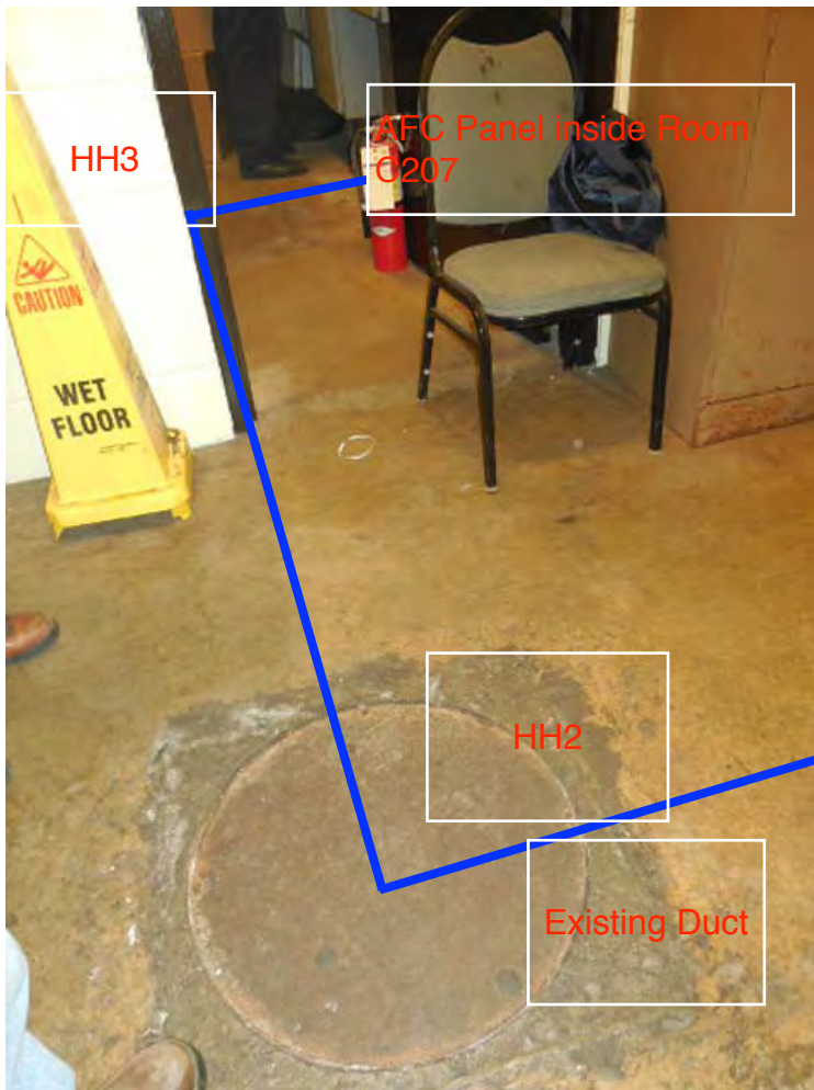
Photo #4: Existing duct route in back rooms.
